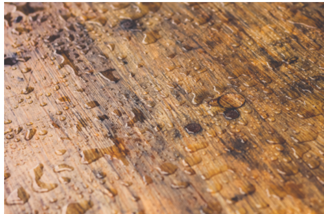
Wood soaked by condensation from high relative humidity.
