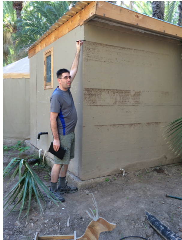
High water mark from flash flooding of the Rio San Ignacio (river Sidon) in Baja California (2014).
